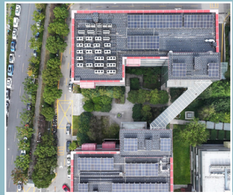
Zhangjiang Data Center in Shanghai
